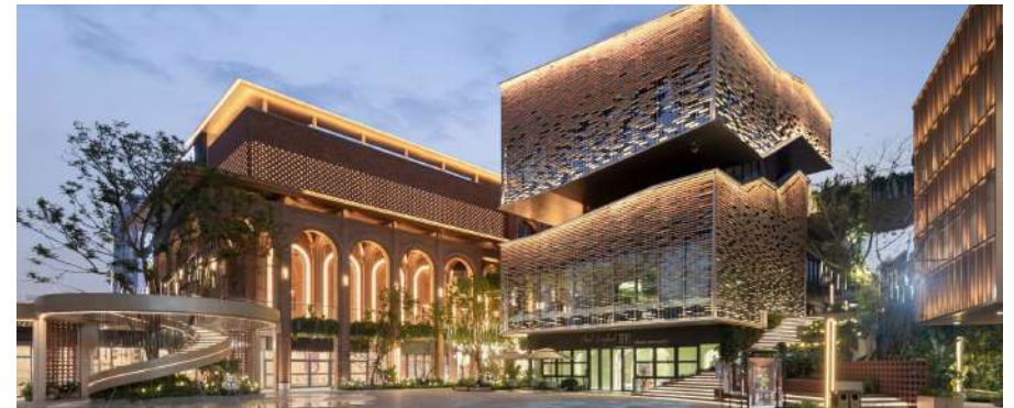
Chongqing Hill - City of Inspiration Chongqing, China
